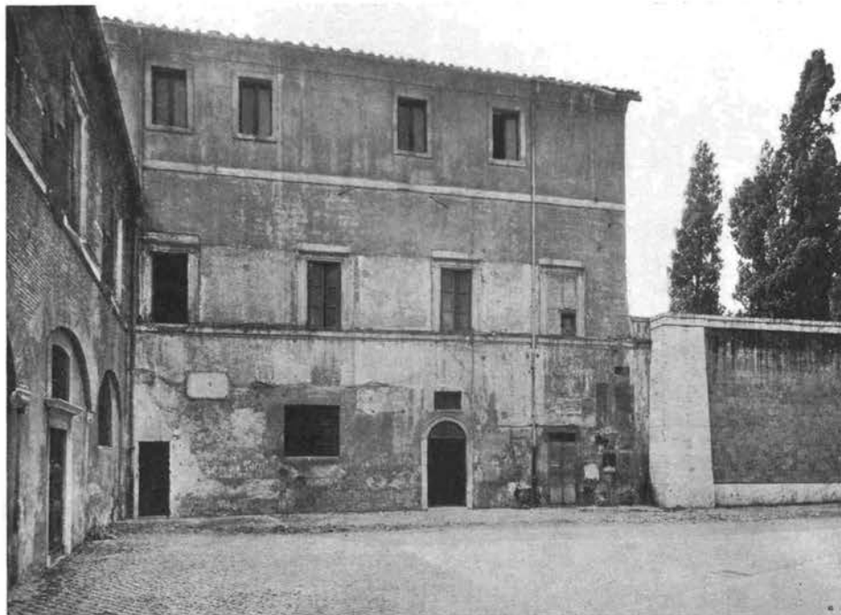
Fig. 96 — S. Lorenzo f.l.m. Convent, west wing from north with northeast corner of basilica maior left of drain pipe (Photo: Sansaini).
